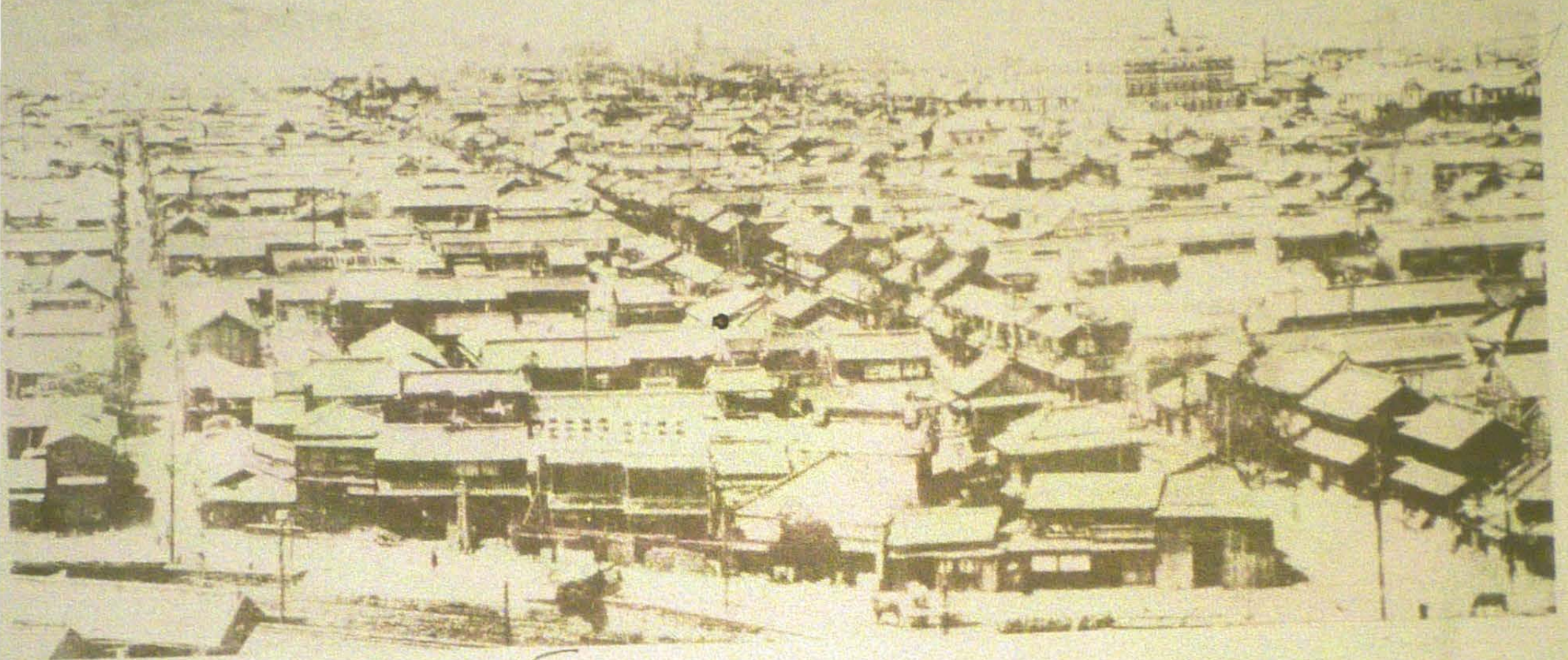
YOKOHAMA. Highly inflammable area, showing lack of fire breaks and large unit fire areas.
