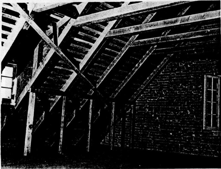
Inside of Tile-Roofed Attic Showing Dormer Window and Masonry End Wall
